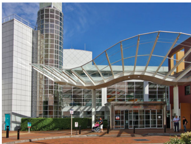
The current entrance to the Children's Hospital at Westmead
