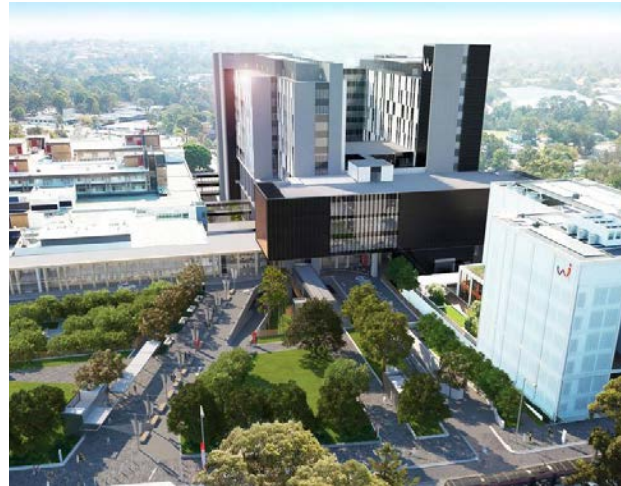
The Westmead Hospital stop will connect patients and visitors to the broader Westmead Health and Education Precinct, including the Central Acute Services Building
